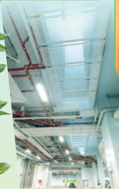
地庫停車場太陽能煙囪系統通風口 Solar chimney ventilation opening in the basement car park
