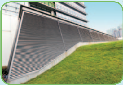
啟德社區會堂天台太陽能煙囪系統排氣口 Outlet of solar chimney on Kai Tak Community Hall roof
