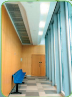
啟德社區會堂走廊的太陽能煙囪系統通風口 Solar chimney ventilation opening in Kai Tak Community Hall foyer
