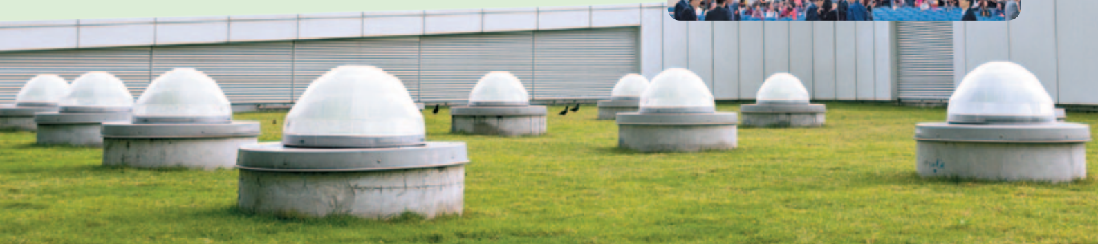
啟德社區會堂天台的日光導管 Sun pipes on the roof of Kai Tak Community Hall
